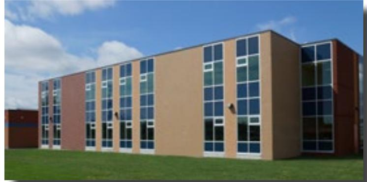
Through a competitive, public bid process, SiteCast Construction and its design team were awarded a design build contract. The tilt-up design leveraged the many cost and time savings associated with concrete construction. This is measured through utilizing insulated architectural concrete tilt-up panels with a thin brick veneer, the elimination of perimeter structural steel, and the reduction in on site interferences and disruptions to the existing student enrolment.
