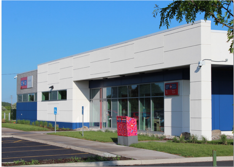
Canada Post Letter Depot-LEED Silver
